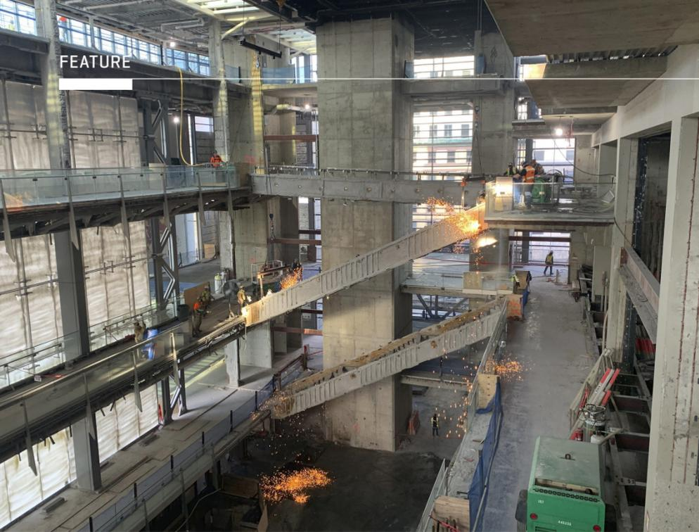
The structural renovation included removing large portions of four floors between levels one through six and replacing the south and east façades.
