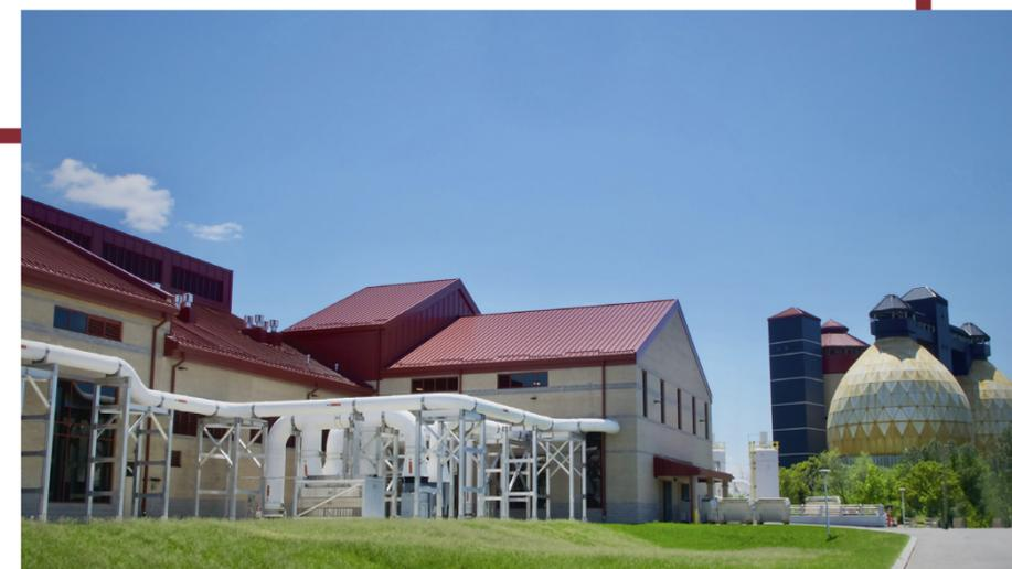
Left: The 45,000-square-foot influent pump station is one of six major structures included in the project's scope of work. The odor control duct is visible in the foreground.
