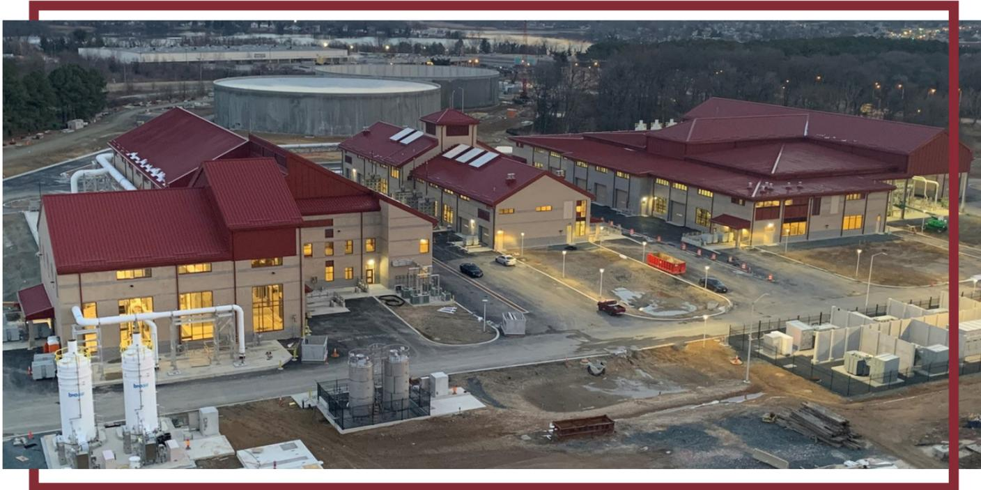
The project replaced the plant's existing headworks to increase influent capacity by 315 percent to 752 million gallons per day. The project also improved screening facilities, pumping stations, and the grit removal process.
